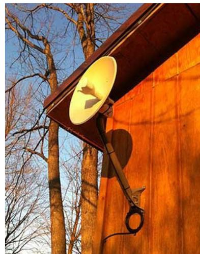
The WISP will install a smaller antenna on the customer's home.
